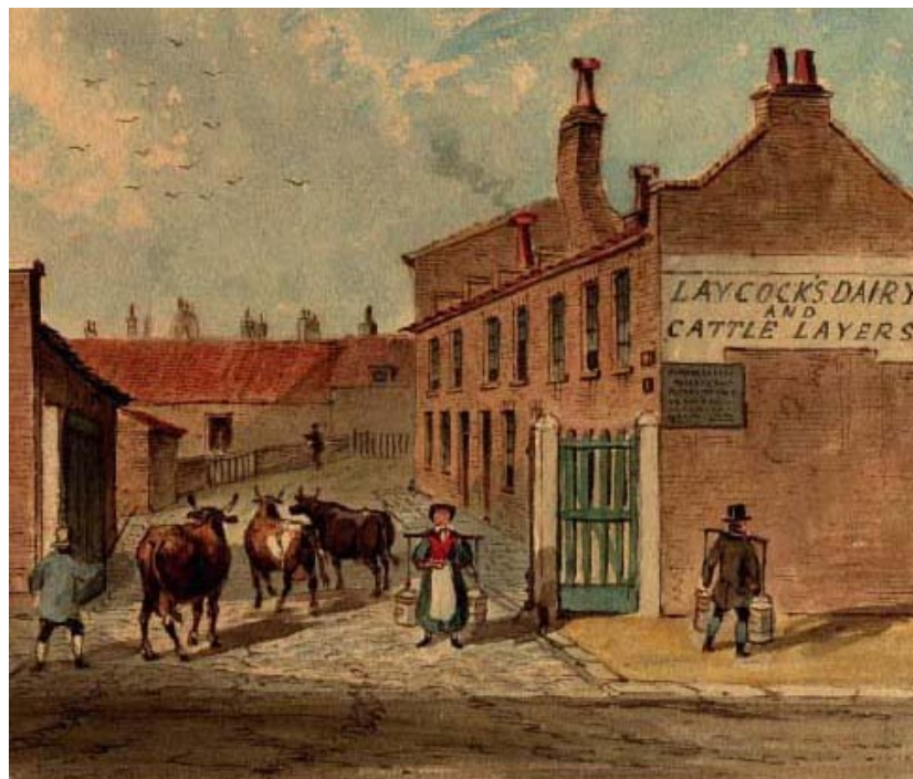
Richard Laycock's Dairy and Cattle Layers (Sheds), c1830
