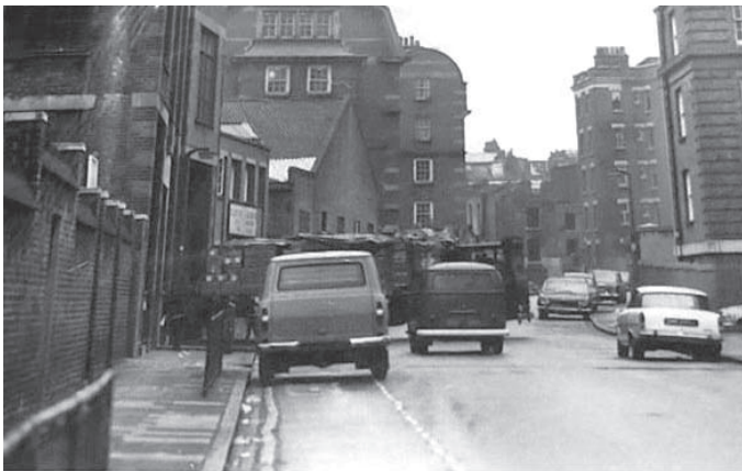
Laycock Street outside Laycock Primary School
