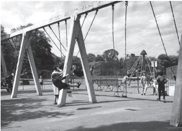
Clissold Park Municipal Swings Installation
