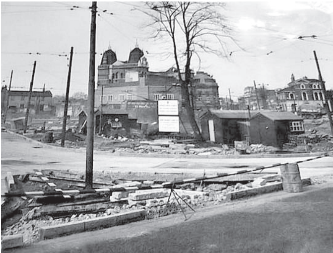
Highbury Corner during Construction of the Roundabout or Gyrotory System, 1958
