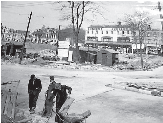
Highbury Corner during Construction of the Roundabout or Gyrotory System, 1958
