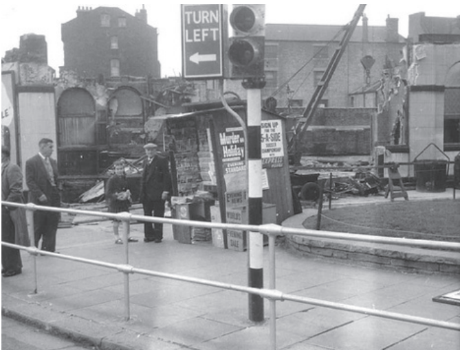
Demolition of The Cock Tavern Remnants, 1956
